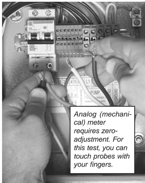
Analog (mechanical) meter requires zero-adjustment. For this test, you can touch probes with your fingers.
