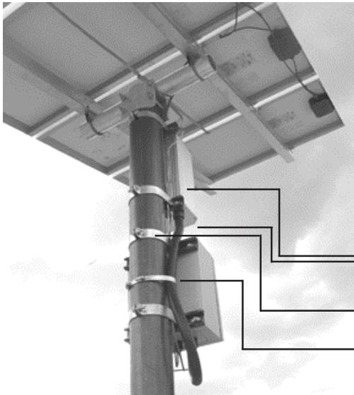
**Typical assembly** of controller and junction box on the solar array mounting pole. Boxes are secured using slotted strut and conduit clamps.
