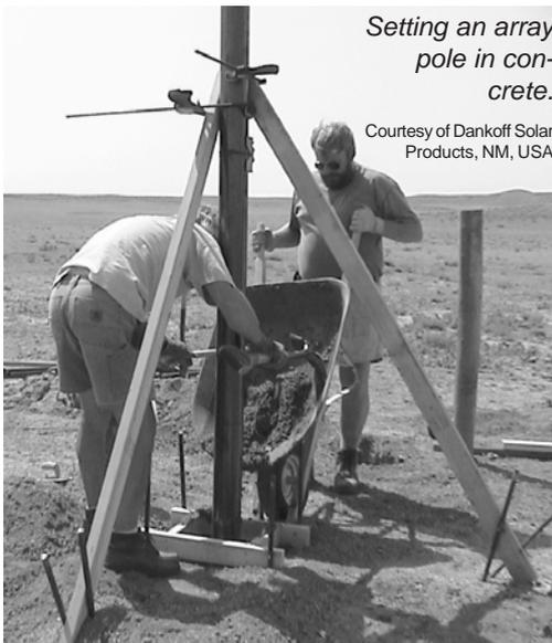
*Setting an array pole in concrete.*
